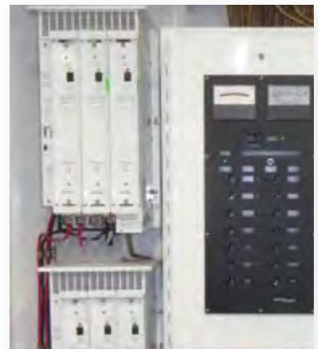
Engine room installation
